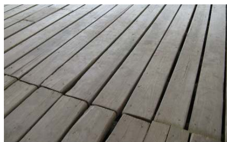
Rustic wooden floor of shed
